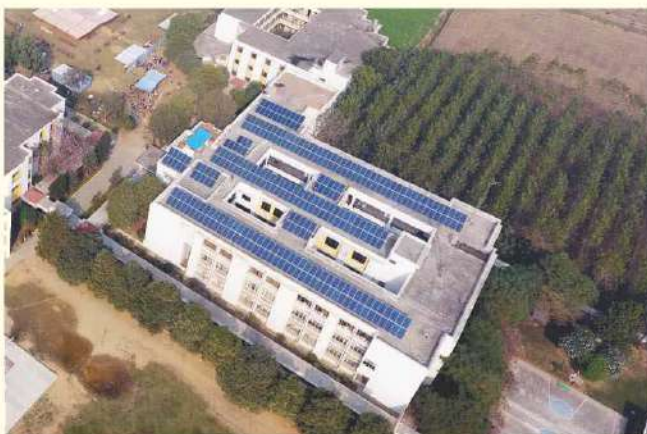
Energy-Saved-Solar Power Plant - 85KW
