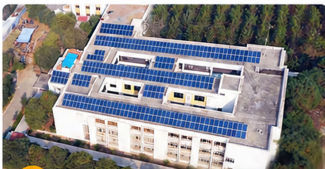
Energy-Saving-Solar Power Plant - 115KW
